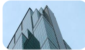
Technical Building Management
